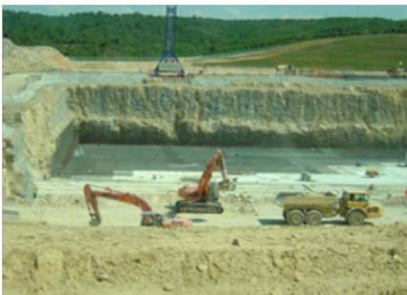
Tokamak pit for ITER, 18 meters deep.
