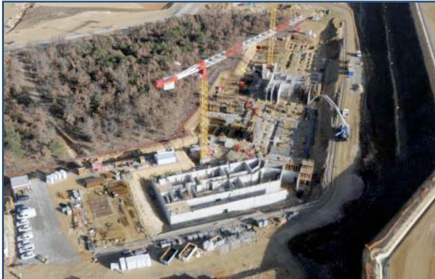
ITER Headquarters Building, under construction. (photo courtesy of ITER)
